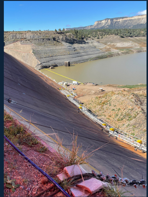
Figure 1: Repairs to El Vado Dam (Built in 1935)
