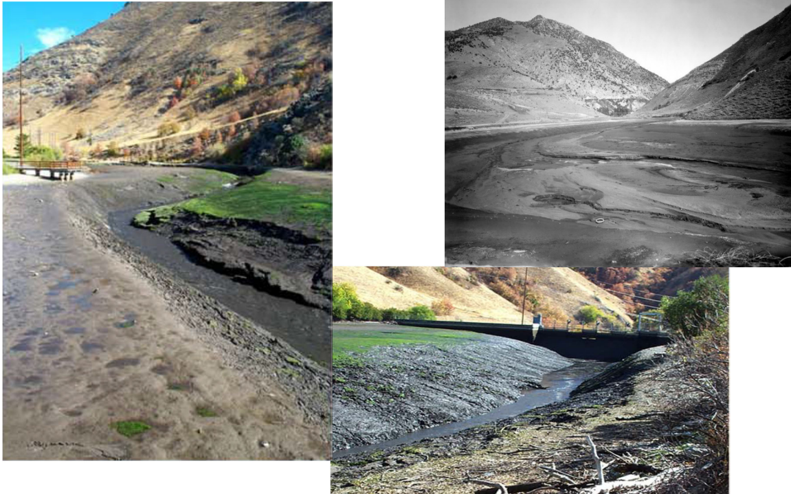
Figure 9. First Dam reservoir, drained. B&W from 1920s, roughly 10 years after dam completed in 1914. Color: October 2001, pool drained to reconstruct dam. Sediment sluicing during low river flow (100 cfs) produced extensive deposition and fish kills downstream.
