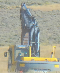
Mobilizing excavator to the Heifer Creek aspen protection project area.
